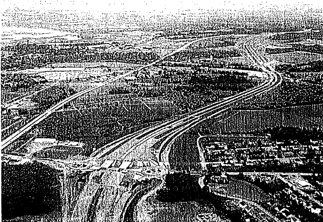
Highway 104 twinning, outside of Antigonish, showing construction of the Trunk 7 interchange, including a roundabout. (Photo courtesy of Ken Wright)
